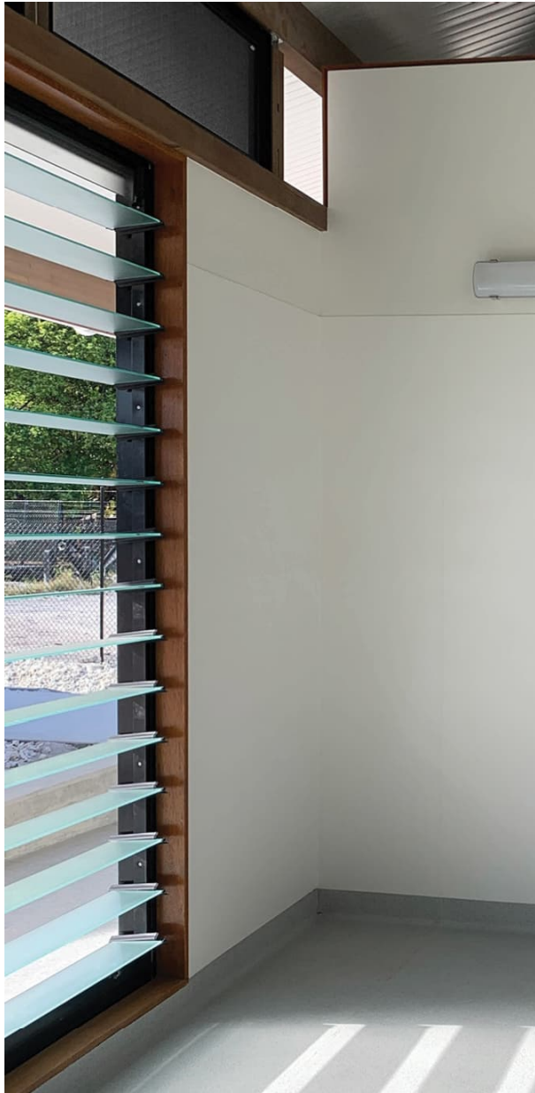
Figure 03 - Operable glass louvers combined with insect screening can be used to promote natural ventilation and passive cooling.
